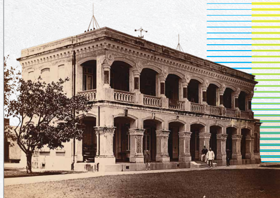
十九世紀末的香港天文台主樓 Building of the Hong Kong Observatory in the late 19th century
