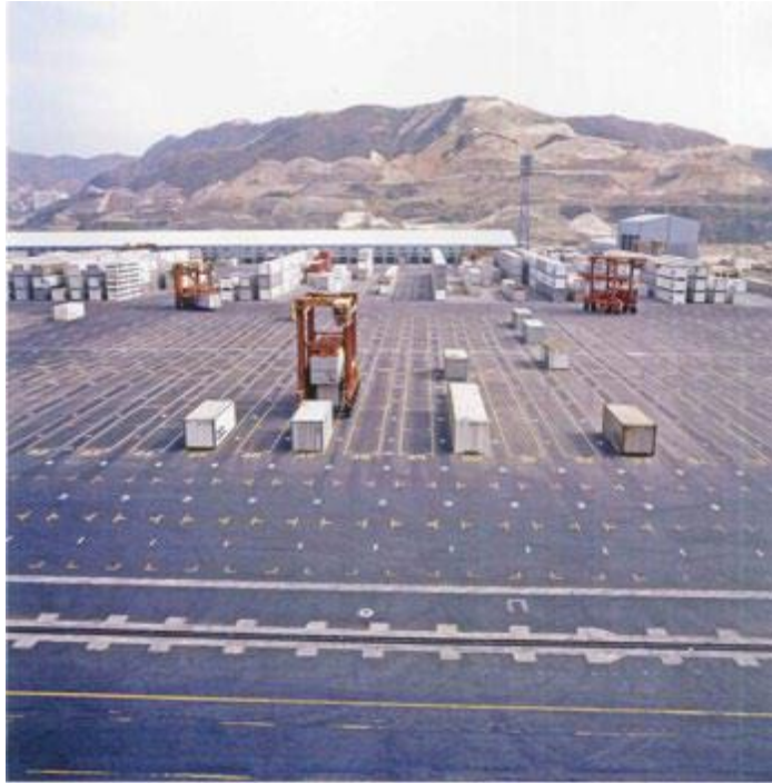
Nicknamed “Monster”, this first-generation hoisting crane was in operation at the Kwai Chung Container Terminal.
