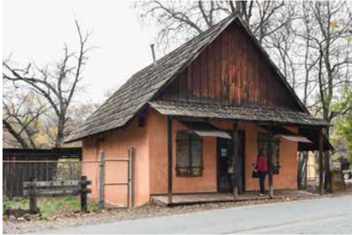
Exterior of the Chew Kee Grocery Store in Fiddletown
